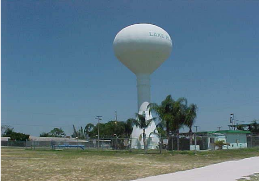
#1 MAGNOLIA WATER TREATMENT PLANT AND ELEVATED TANK
